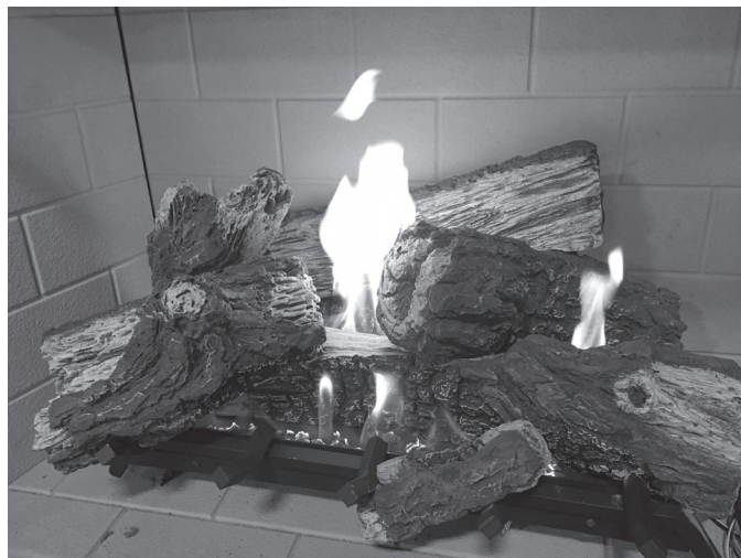
Figure 6.13 - Correct Appearance of Rear Flames
